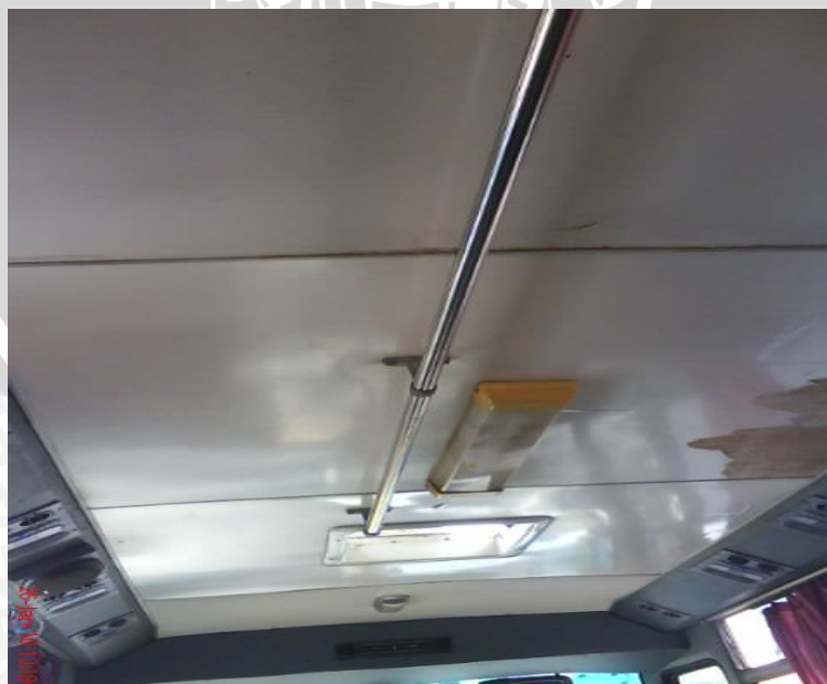
Gambar 4.13. Kondisi Langit-Langit Bus
