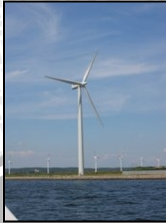
Gambar 2.4 Turbin angin modern di Denmark Sumber: wikipedia , 2009
