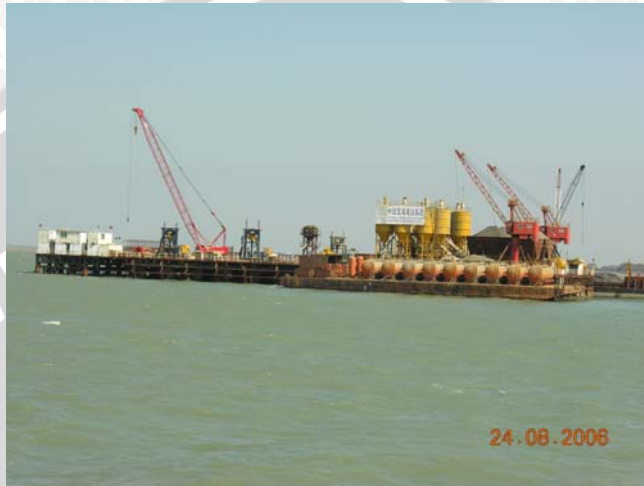
Gambar 2.3 Auxiliary platform dan platform pengecoran (Dok. PT. LAPI ITB)
