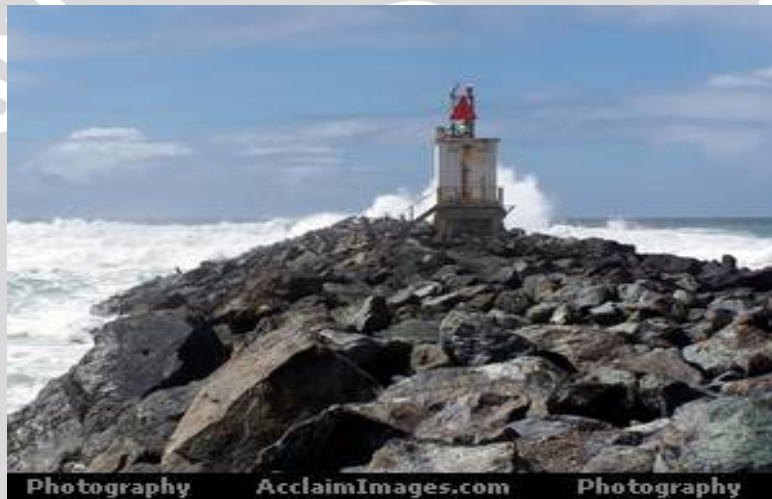
Gambar Struktur Rubber Mound Revetment
