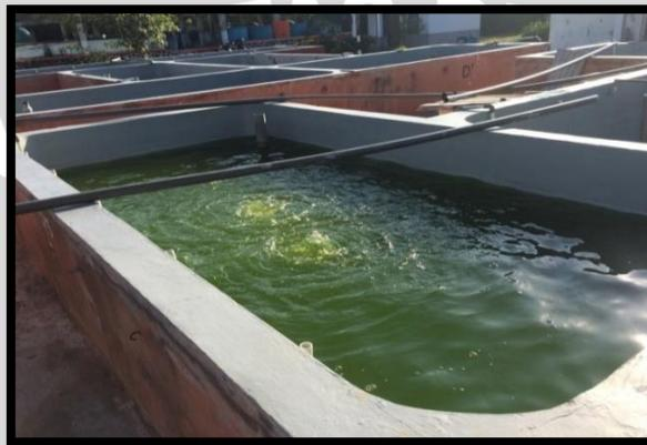
Gambar 3. Bak Beton Massal
