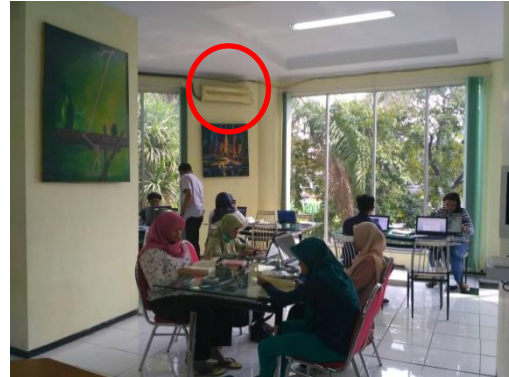
AC split wall
