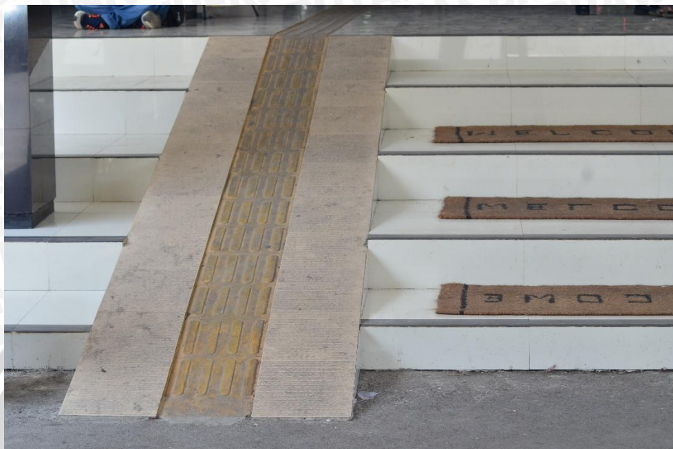
Gambar 20. Lantai Miring/ Ramp Permanen
