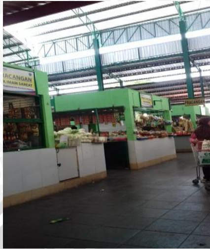
Gambar 6 : Kondisi Interior Pasar Oro-Oro Dowo
