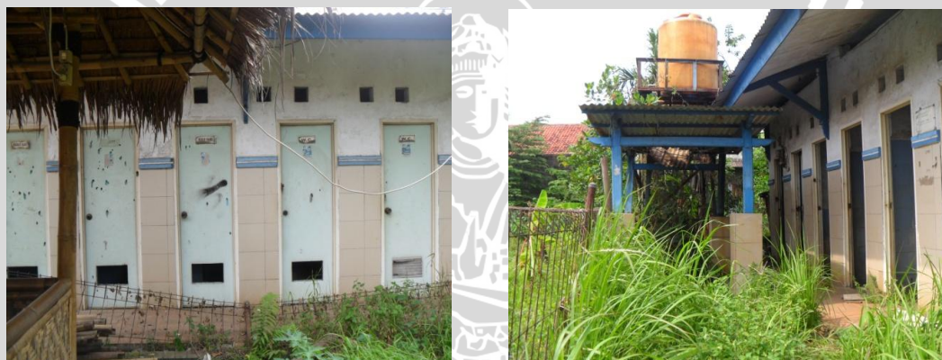
Figure 19. MCK Rawabali Which has Inactive And Not Maintained Anymore In The Kelurahan Mekarsari
