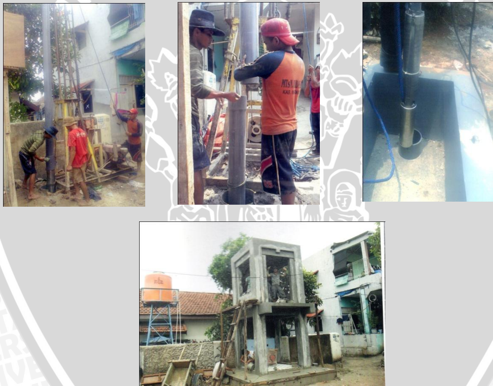
Figure 16. Process of Water Wells Construction and Building In The Kelurahan Jatiuwung Kecamatan Jatake by Dinas Pekerjaan Umum Tangerang City (Source: Documentation of Dinas PU Tangerang City Activities, 2013)
