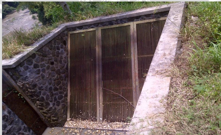
Gambar 9. Trash Rack
