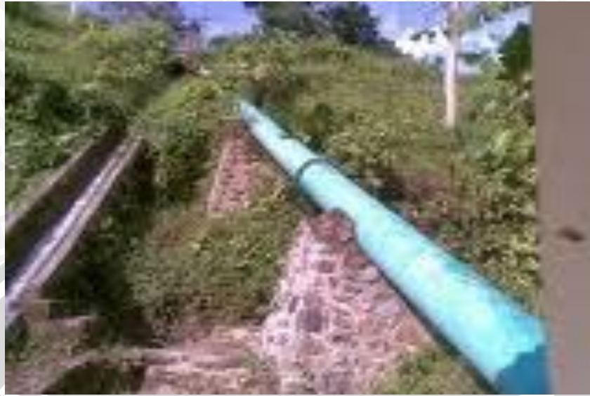
Gambar 10. Pipa Pesat ( penstock )
