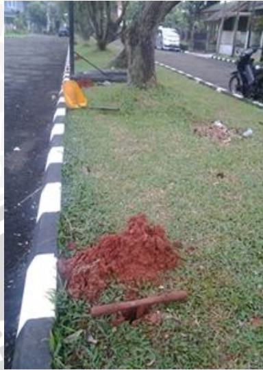
Figure 9. Biopori Holes in Progress Source : Documentation at Flamingo Cluster, Sector 9, 12 th April 2014
